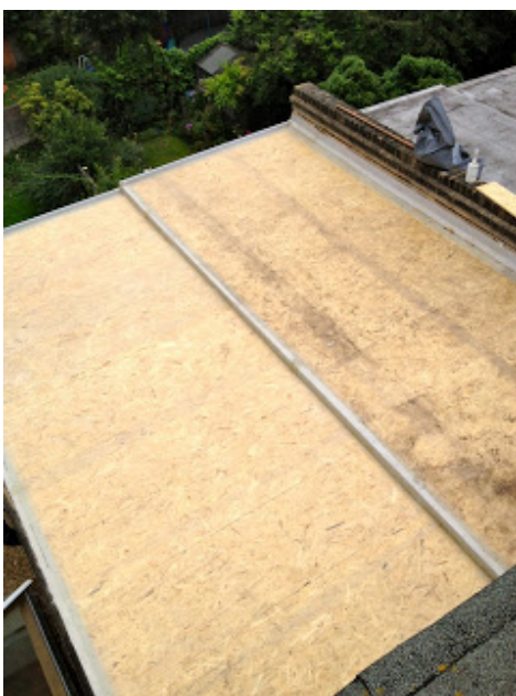
New deck with GRP system (pre resin)
